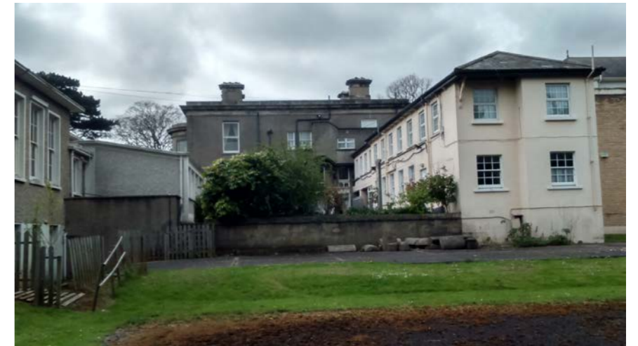
North elevation addressing Temple Road with former structures in place
