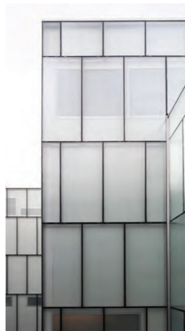
OPAQUE GLASS BACKING PANEL TO PENTHOUSE FACADE
