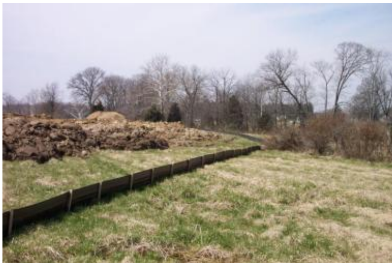
Figure 5 – Typical silt fence
