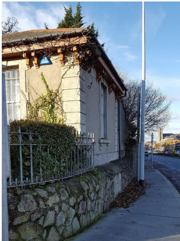
Figure 17.10 - New boundary wall
