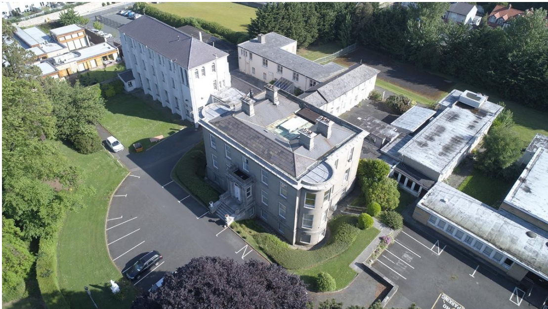
Figure 17.6 - Aerial view from South (pre-2021 demolitions)
