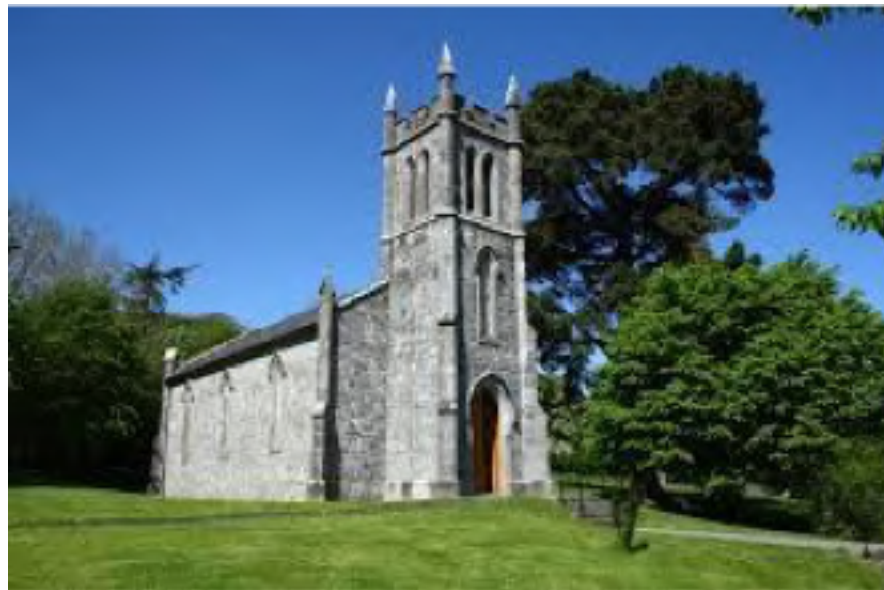
Figure 25 - Ardcroney Church Originally from Tipperary, now in Bunratty Co Clare
