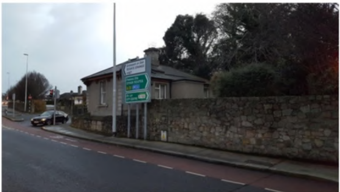
Figure 5 - Gate Lodge fronting on to Temple Hill
