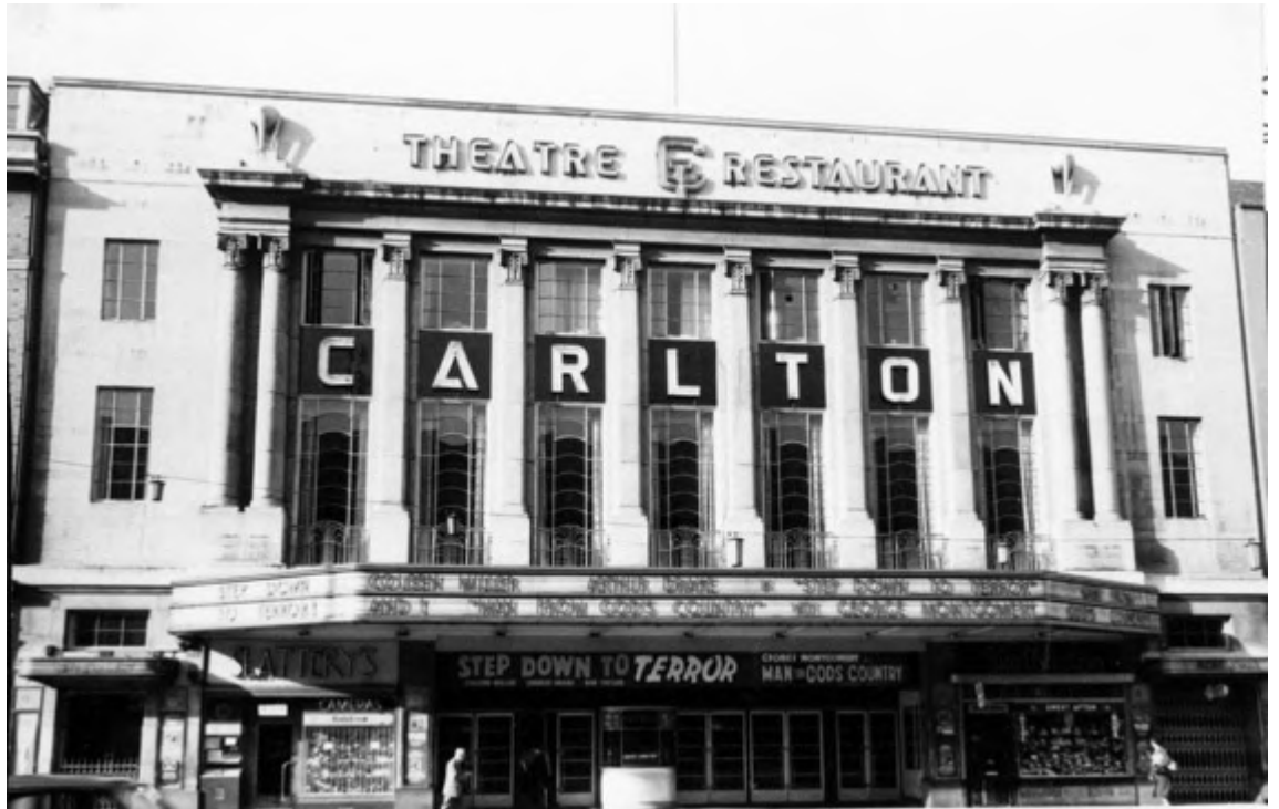
Figure 17 - Carlton Cinema Façade O'Connell Street Dublin
