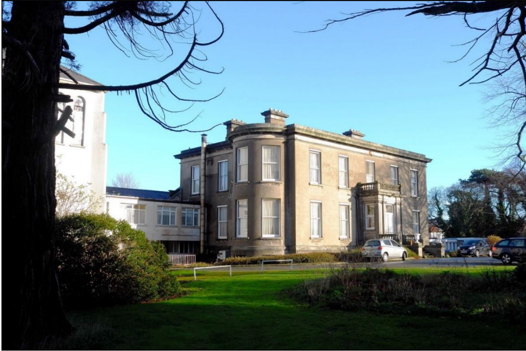
Plate 16.1 St. Teresa's House from the southwest
