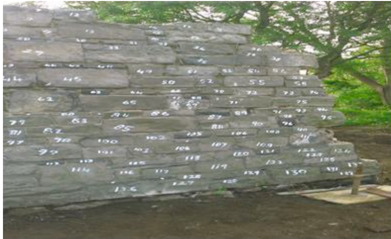
Recording prior to deconstruction. Photo courtesy of Nolan Conservation
