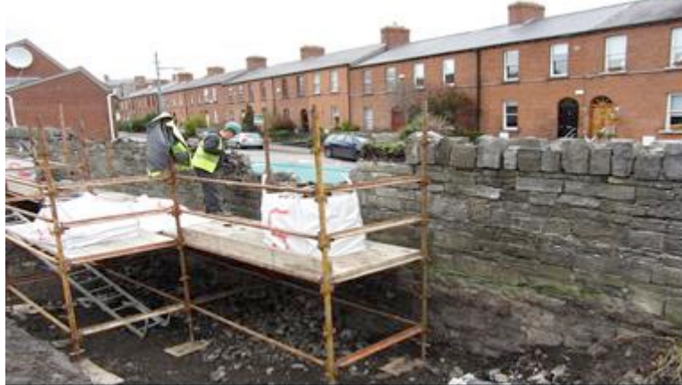
Rebuilding of wall Photo courtesy of Nolan Conservation
