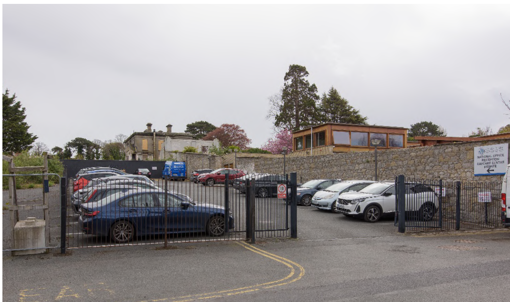
Figure 13.4 – A view of Craigmore House from the access road to the neighbouring Alzheimer Society office
