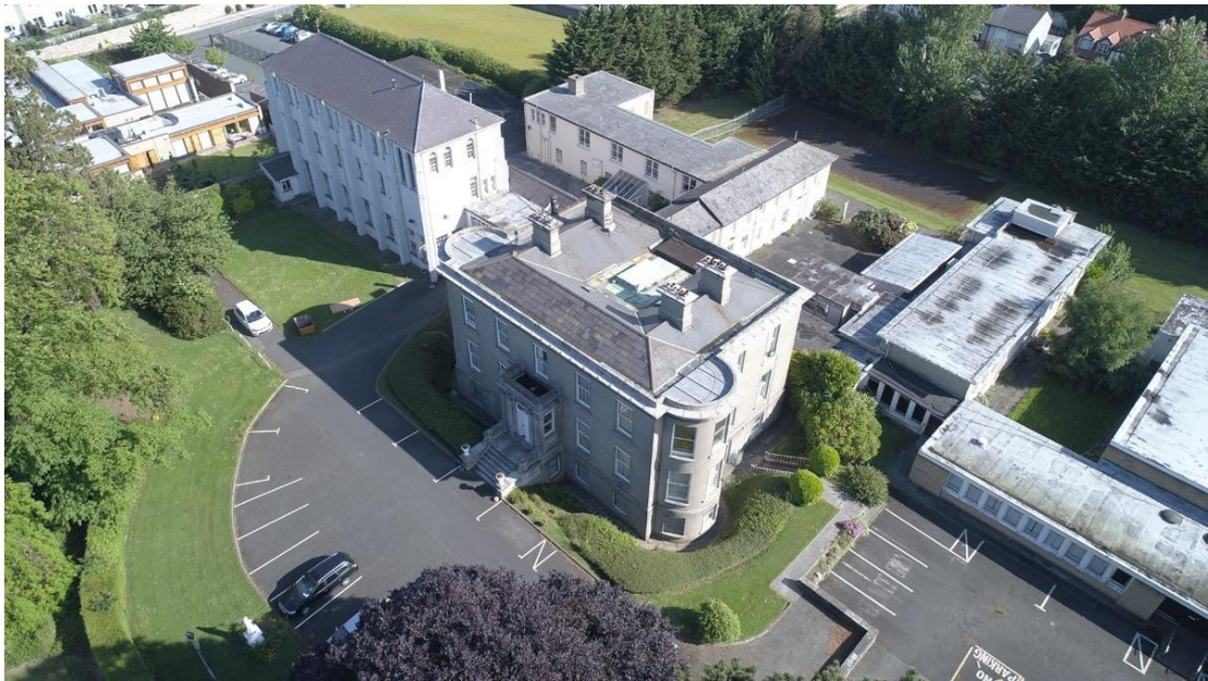
Figure 17.6 - Aerial view from South (pre-2021 demolitions)
