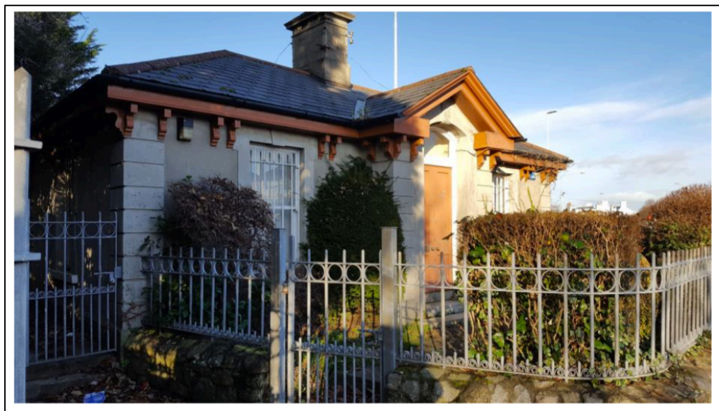
Figure 2.3 - Front of the Gate Lodge
