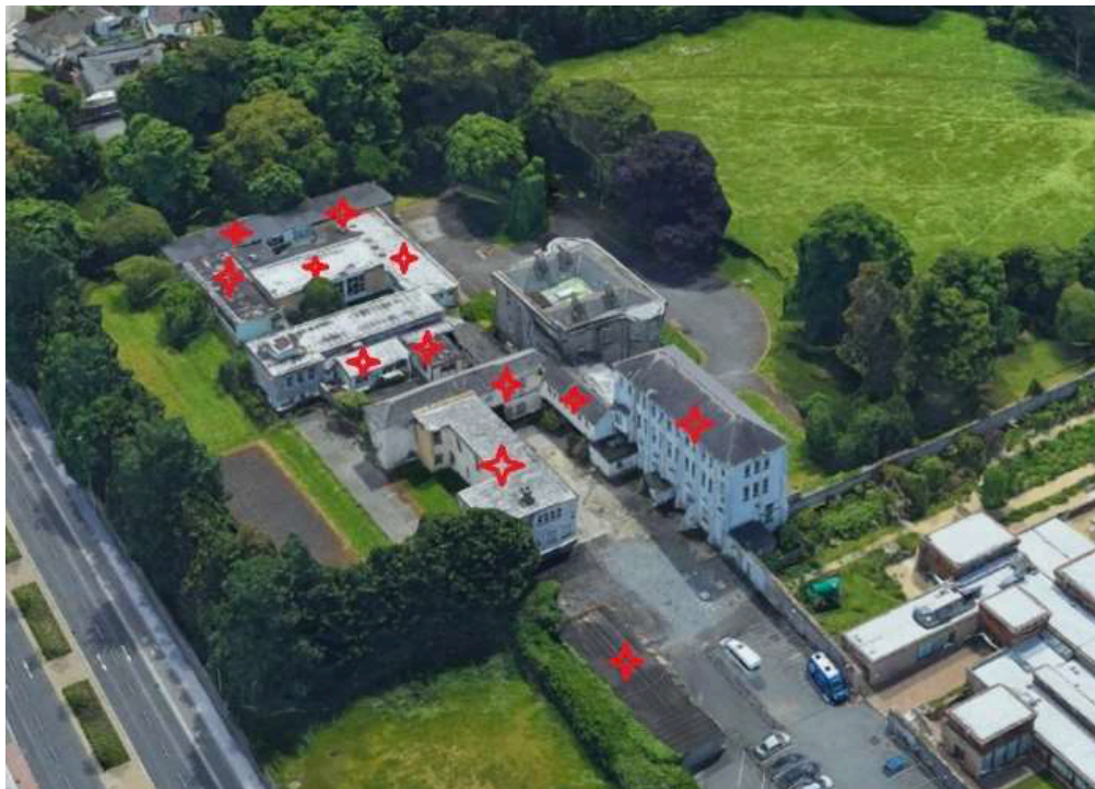
Figure 2.5 Google Earth view of buildings demolished as indicated with the red stars.
